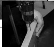
Make sure to drill the holes perpendicular to the shutter so as not to break through the surface of the shutter.
